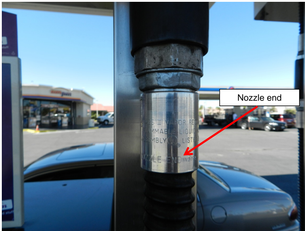
Photograph # 3: Nozzle # 20 hose with nozzle end connection attached to the breakaway coupler.
